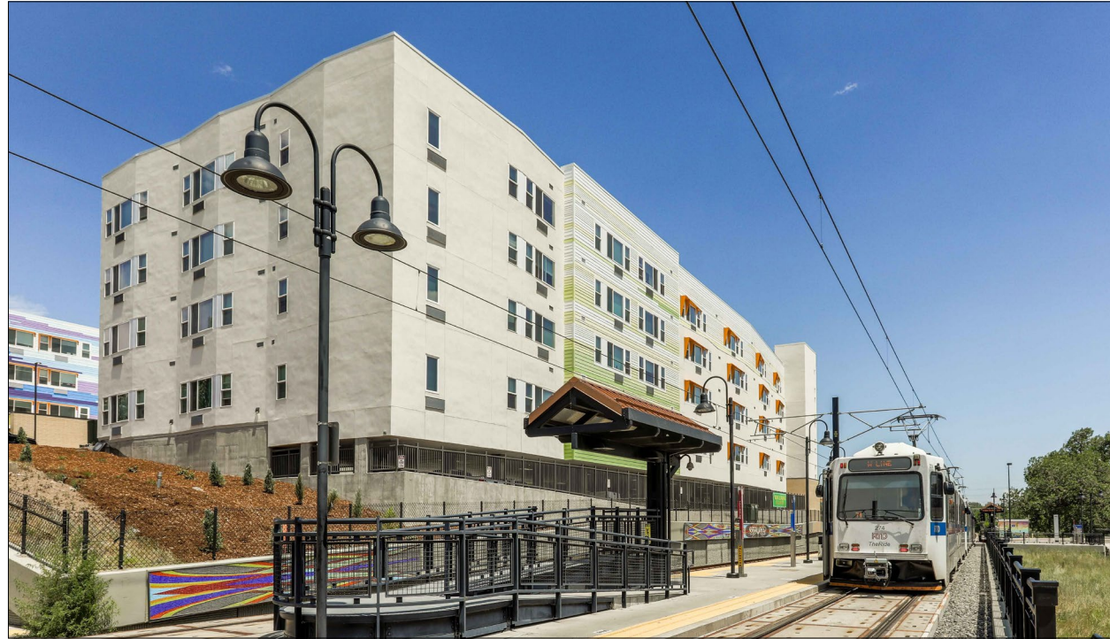
Arroyo Village, which received a $750,000 AHP grant, brought much needed affordable housing options to West Denver.
